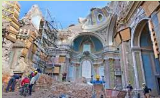
Failure of monument after the 2009 L'Aquila Earthquake (S. Maria di Paganica)
