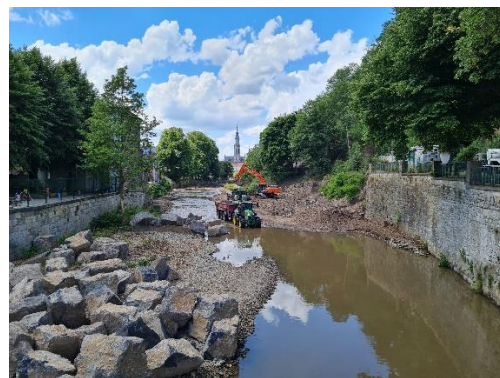
Repair works in the riverbed, Vesdre valley, Belgium
