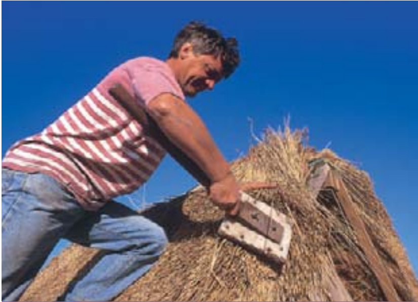
A roof being thatched in Brittany (France)
