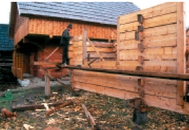
Wooden houses are still being built using the same techniques as in the past: the building is laid out in pieces on the ground and then assembled from the base upwards
