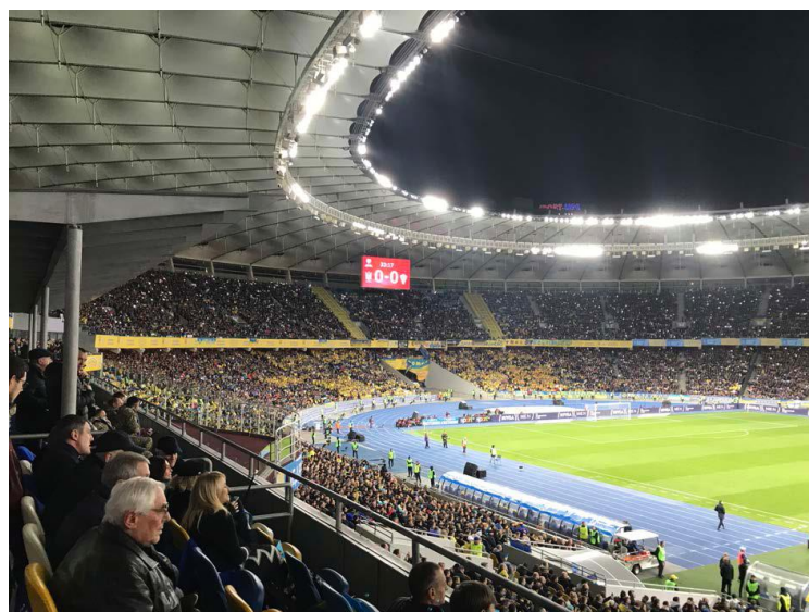
Picture 12 - Segregation netting next to vomitories compromising (emergency) exit capacity
