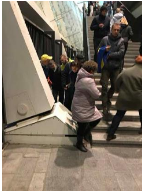
Picture 26 – Fans using unsafe shortcut between stairs and structural columns
