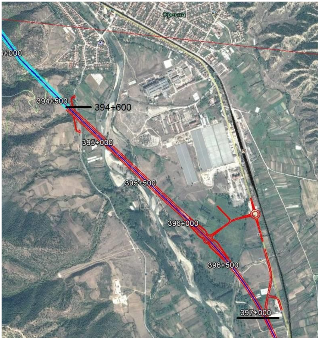
Figure No. II.1-7. Situation of the road section, km 394 + 605 south portal, right roadway of Kresna tunnel, km 394 + 600 south portal left roadway of tunnel Kresna, end of route 397 + 000, where it enters Lot 3.3.
