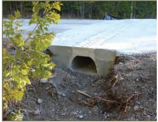
Photo 30. Earth excavated to allow at grade entrance to tunnel. © D. Filip
