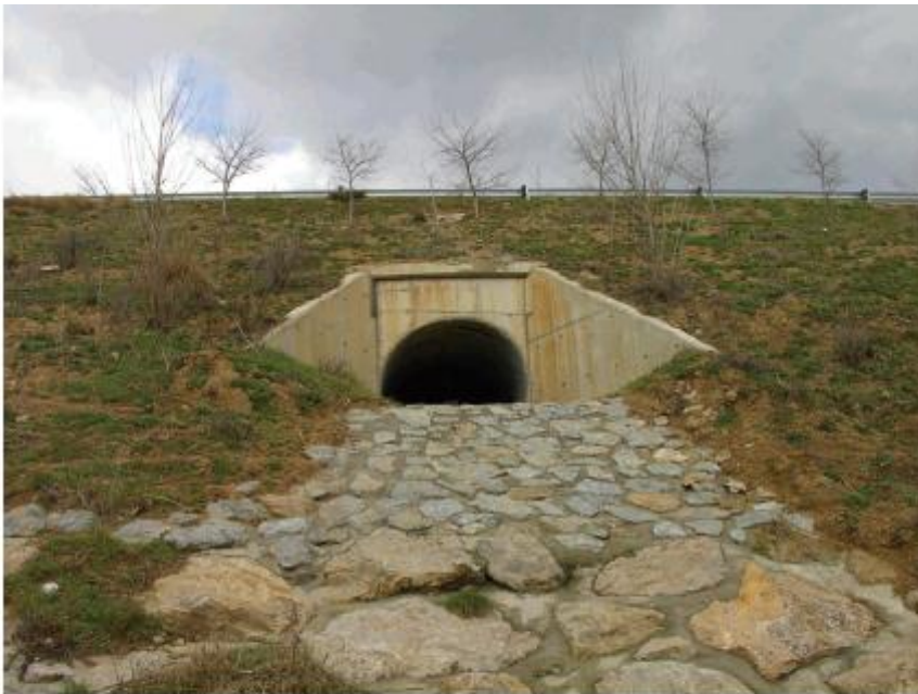
Figure 7.64 - Stepped exits of drains are traps for small animals (top). The two exits in Spain (centre, bottom) have been adapted so that animals passing through the drainage culverts do not get trapped. (Photos by C. Rosell)
