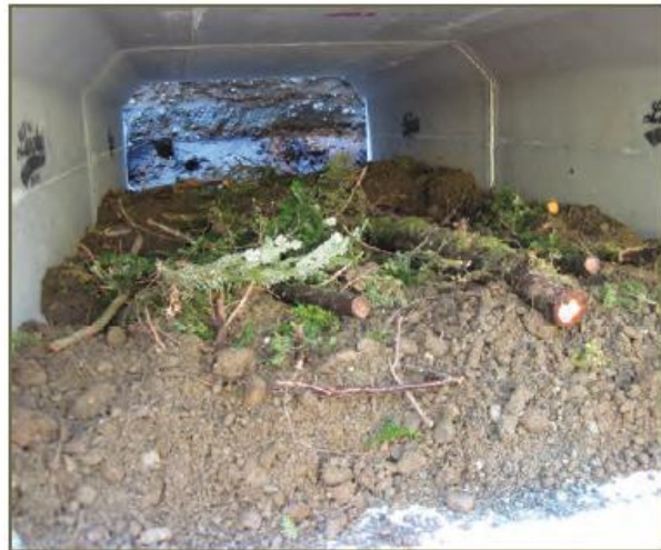
Photo 13. Soil and branches inside tunnel bottom, Ucluelet, B.C. ©Barb Beasley
