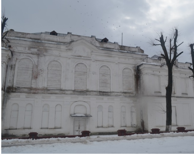
Mscislaŭ. Former Men's Gymnasium Building. View from the Jesuit College
