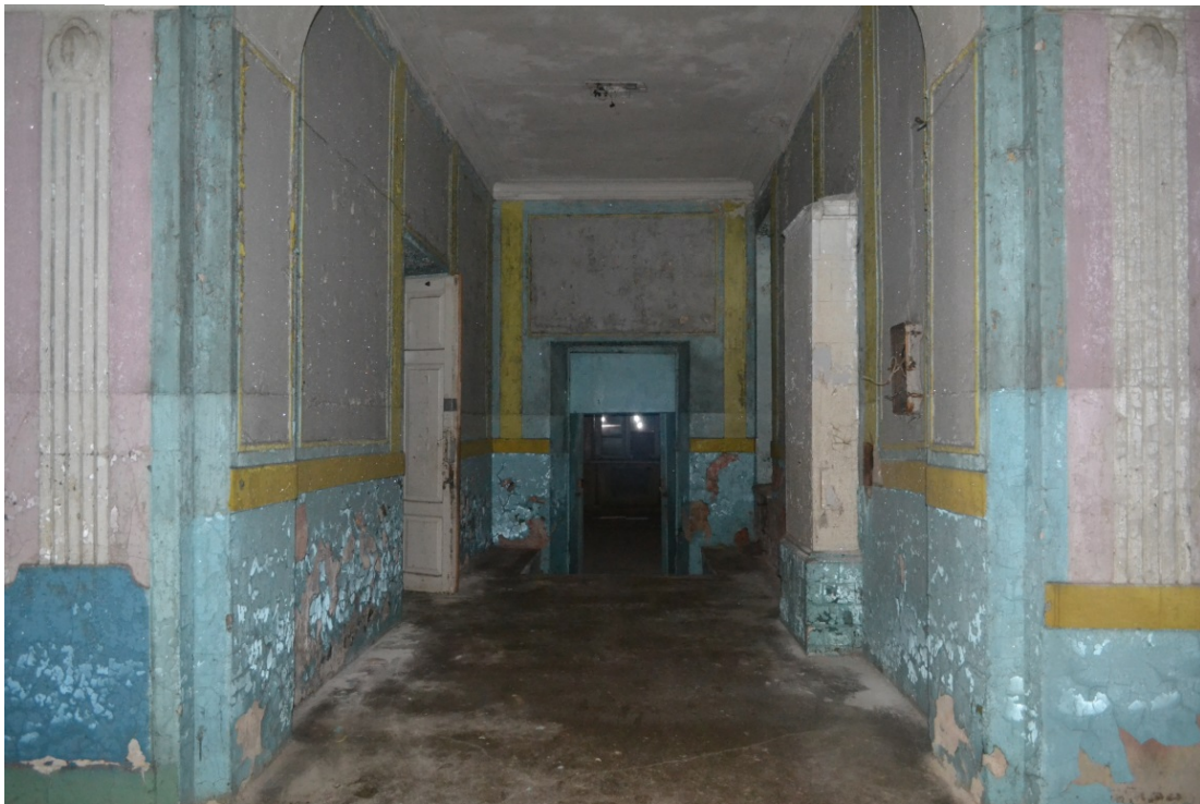
Mscislaū. Former Men's Gymnasium Building. View of the interior.
