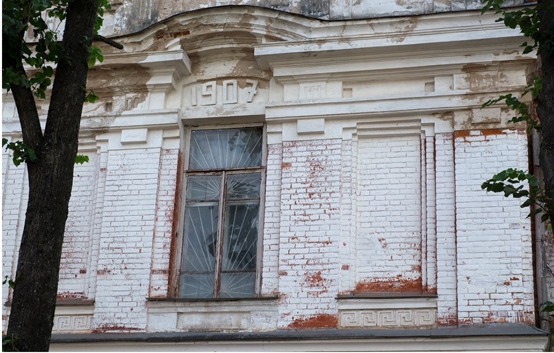
Mscislaū. Former Men's Gymnasium Building. View of the façade.
