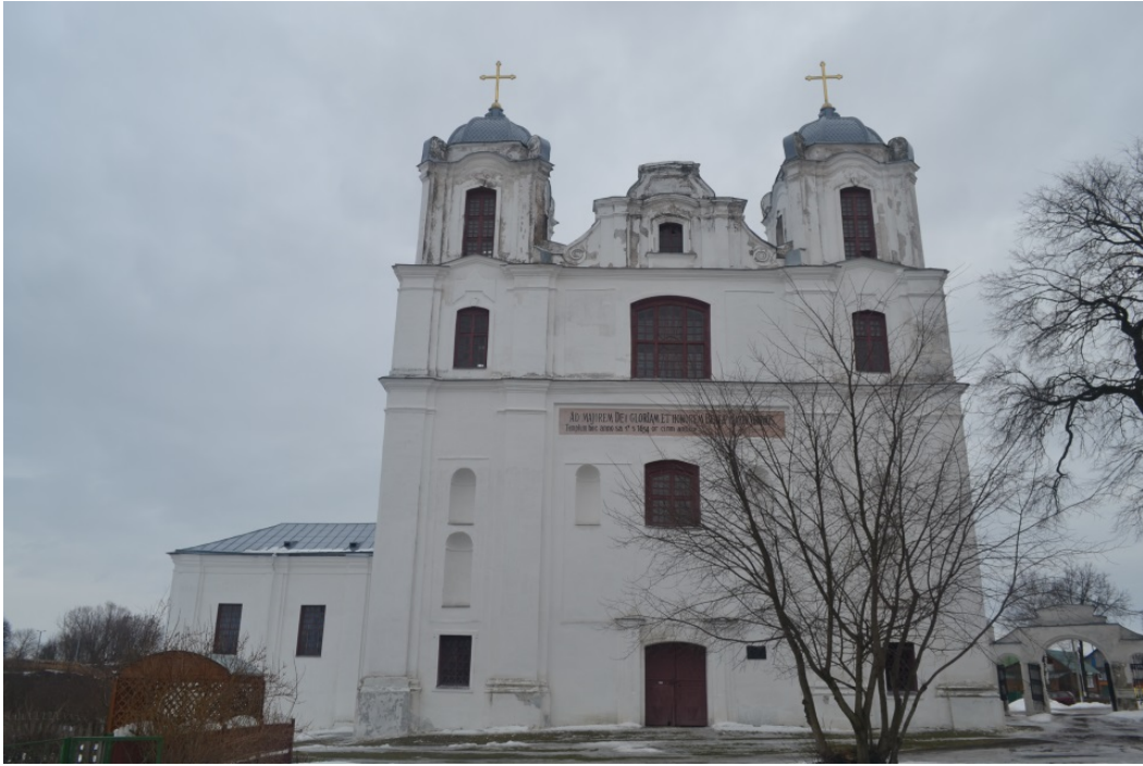
The Carmelite church. View of the west facade of the church
