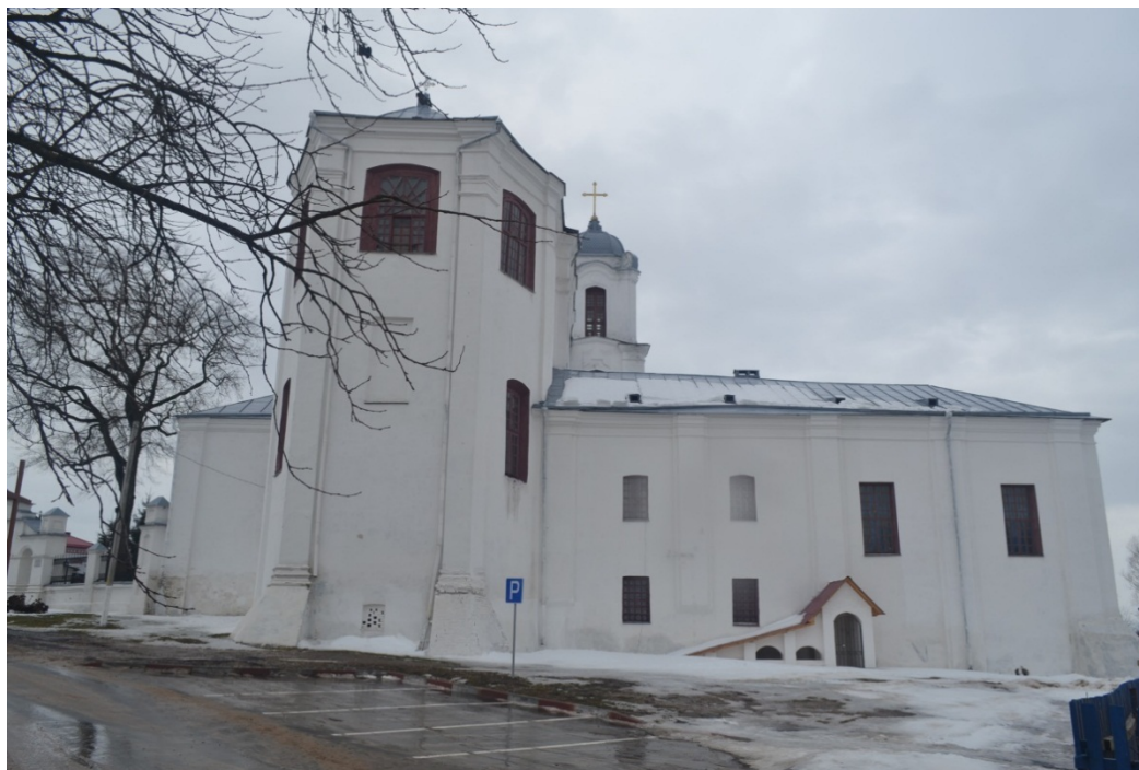
The Carmelite church. View of the east facade of the church from the side of the car park
