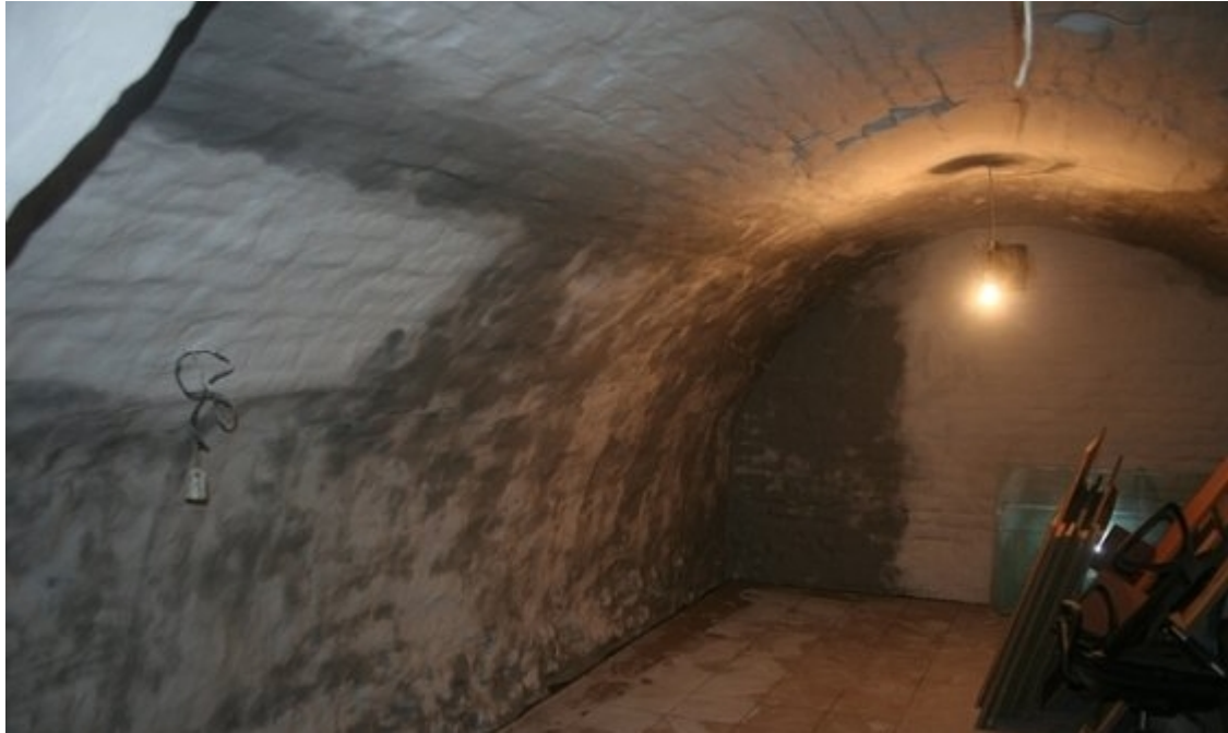
Cellars of neighbouring house to Town Hall on Market Square
