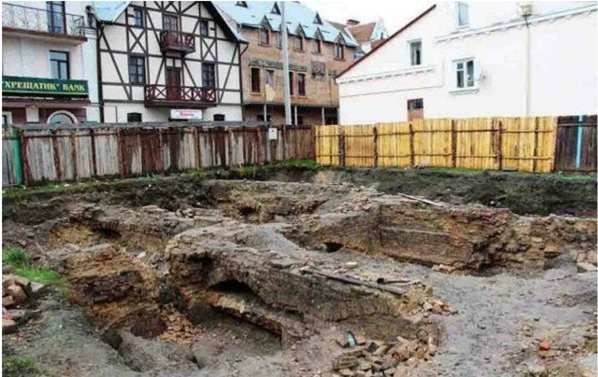
Destroyed, cellars in the Old Town
