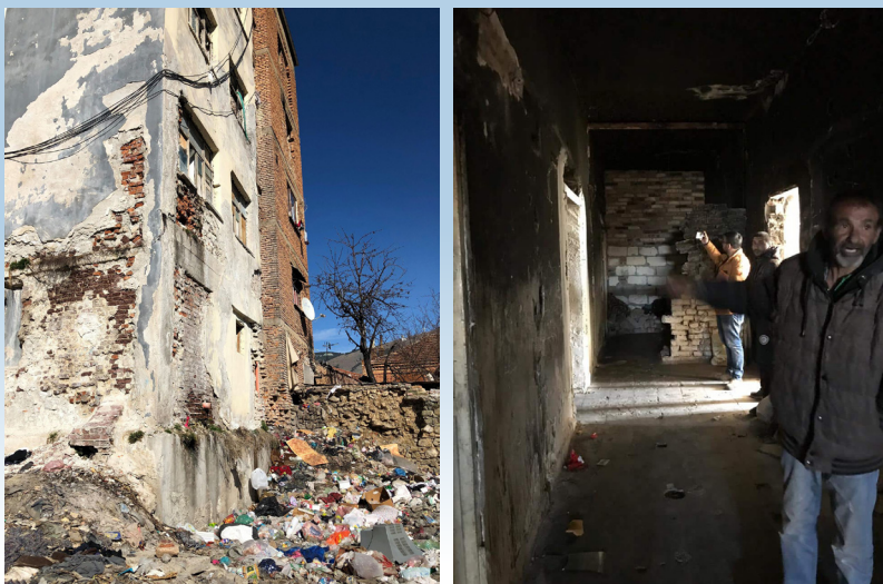
Figure 2. Pictures from field visits (former dormitories)
