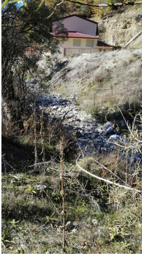
Photo taken above powerhouse, Nov 2, 2017
