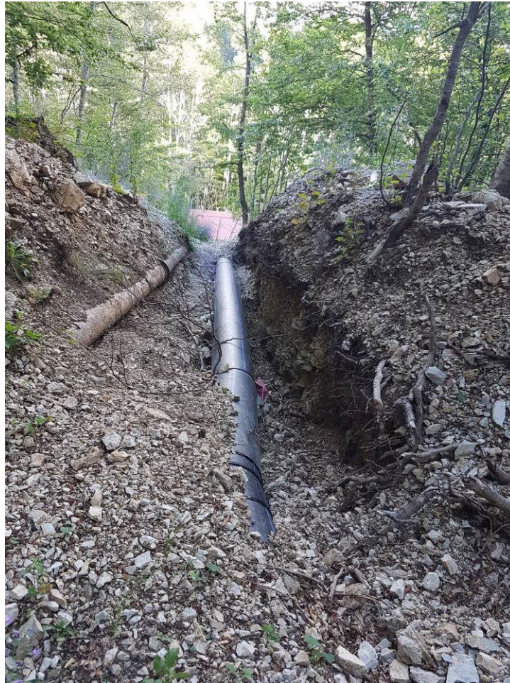
HPP on Kakachka River, pipelines, NP Mavrovo
