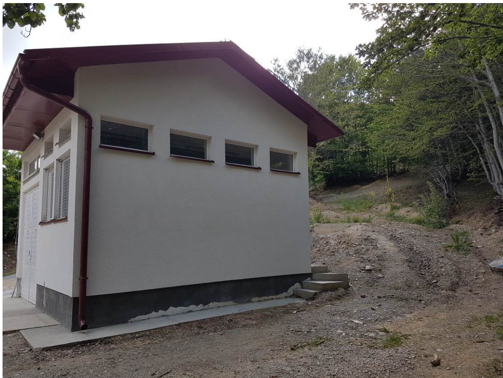
HPP on Belichica River, Powerhouse, NP Mavrovo, no remediation of surrounding area
