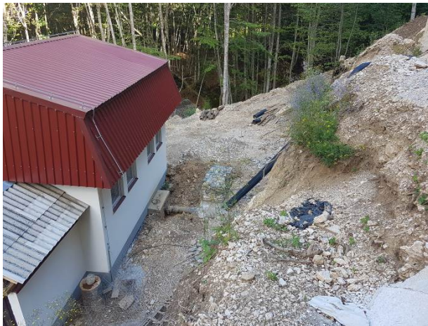
HPP on Kakachka River, powerhous, NP Mavrovo, bad construction practice
