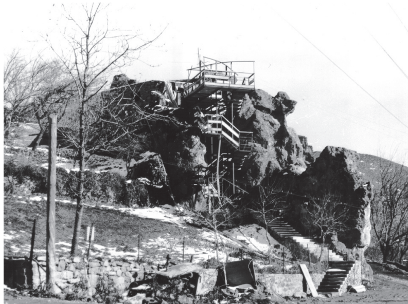
Picture 10. Residential Cavern
