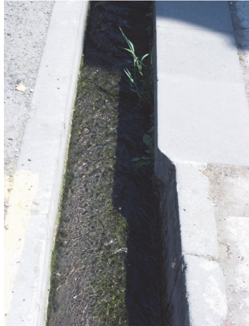
Picture 14. A Restored Water Channel
