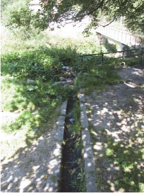
Picture 11. Water Channel, River Pouring Section
