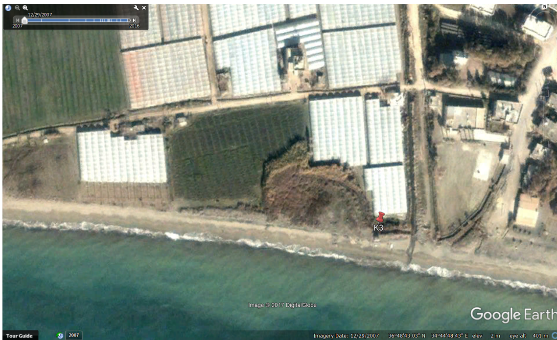
Figure 1: coastal erosion progress (Google earth aerial photograph, 2007)
