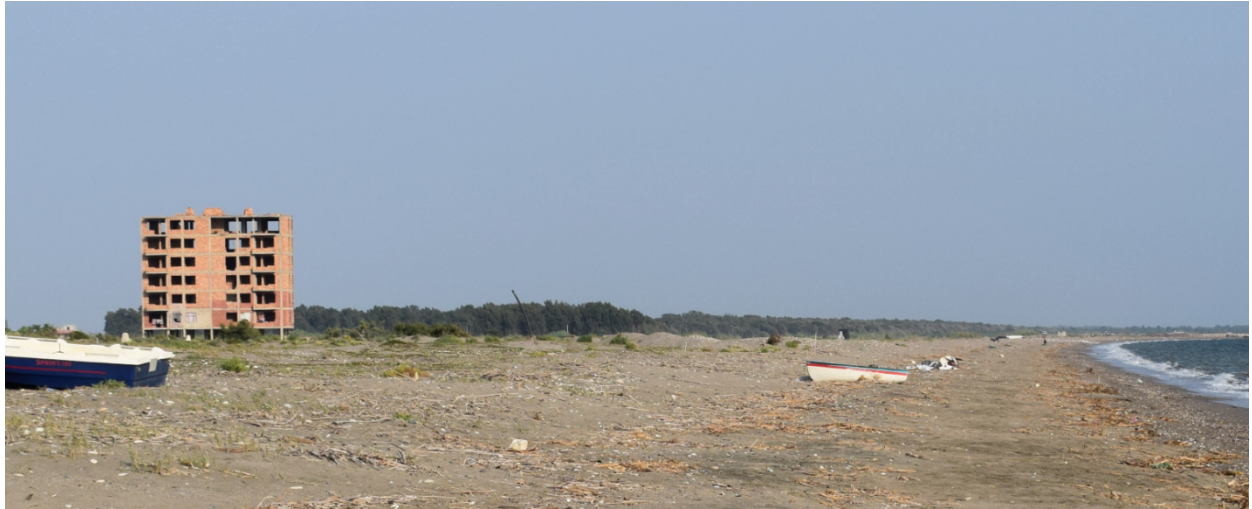
Figure 27: abandoned building in beach section K1
