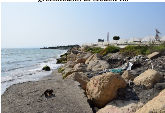
Figure 5: rocks at the beach in front of greenhouses in section K3
