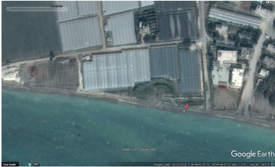
Figure 2: coastal erosion progress (Google earth aerial photograph, 2017)
