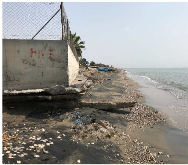
Figure 21: The erosion of the coastline effecting the concrete wall of the local school yard.
