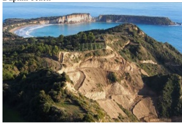
Photo 12: The illegal road construction in the area between Daphni and Gerakas.
