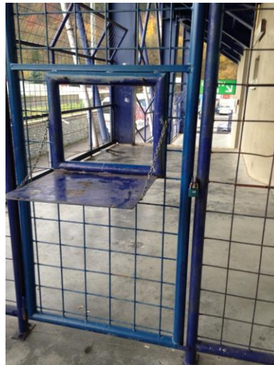
Service hatch for refreshments for visiting supporters
