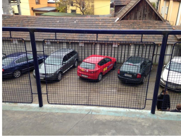
Barrier and guarding at high level in main stand
