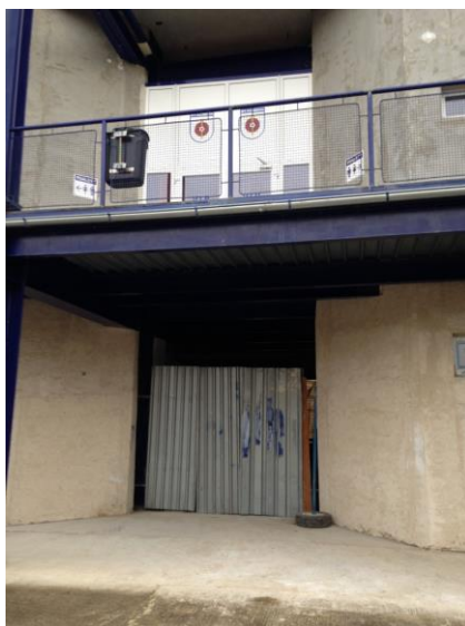
Disused area under main stand
