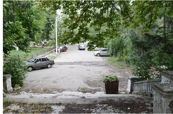
The square in front of the former Zemstvo building is deteriorated and used as parking
