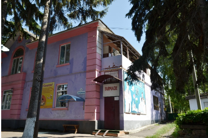
Example of intervention on a historic building on street M. Kogalniceanu, - the facade was painted in inadequate colors, the original carpentry has been replaced with PVC windows; part of the facade is covered with billboards
