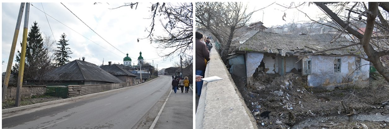
Extending Stefan cel Mare street over the brook Racovăț left existing houses at a lower level without road access. Many of them are ruined or abandoned.
