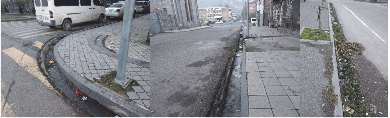
Figure 3 - Stormwater collection system
