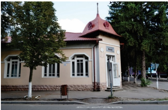
The Balter Pharmacy, façade from Independenței strada
