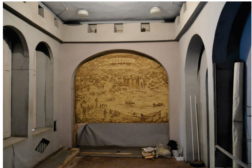
Inside the building – plasterboard plates were placed on the walls
