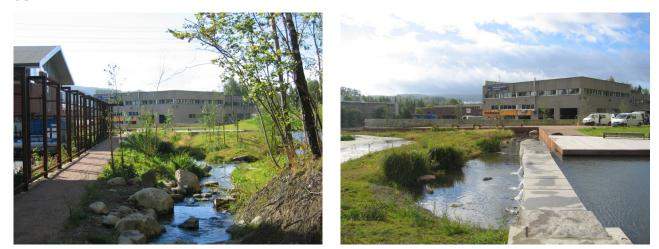
Left: At the top end of the area, the river water is channelled into the water park through a narrow section, with a walking path along the side. Right: The water park is divided into two levels, with a dam at the top end and a wetland at the bottom end. (Photo: I.H. Kjerkreit, 2007)
