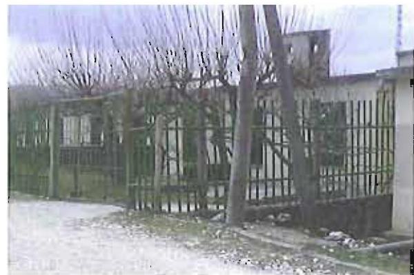
View of the pumping stations
