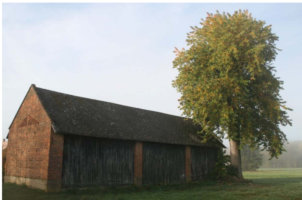
Barn of traditional style and hold-over maple specimen in Bödeháza, which were included in the cadastre of unique landscape assets of the village
