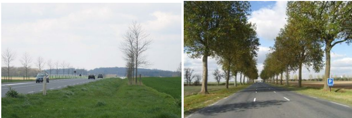
Figures 21 and 22: Even when the local authority decides to bear the additional costs involved in land acquisition, excessive planting distances make it impossible to re-create the “cathedral” effect produced when the proximity of the road and the trees creates a distinctive and integrated space.
