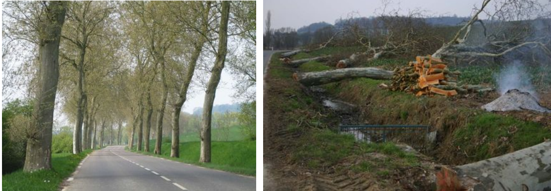
Figures 68 and 69: The ditch exposed after cutting down this double row of plane trees is not designed to mitigate accidents. In France, ditches, along with embankments and rock faces, constitute the solid obstacle accounting for the largest number of serious injuries and the second largest number of road deaths.
