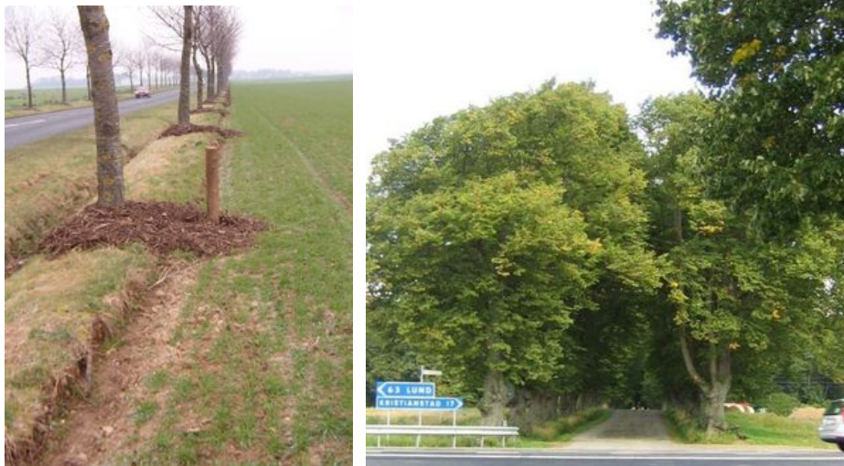
Figure 106: Posts used to protect trees from damage in France. If the trees had been planted on the verge, between the roadway and the ditch, the risk of impact damage would have been minimised while at the same time restricting root growth in the direction of the cultivated land. Figure 107: A strip of fallow land – here in Sweden – provides protection against impacts and soil compression.
