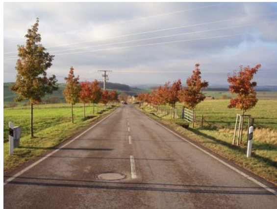
Figure 102: Young pear trees spaced at distances gradually reducing from 15m to 10m to signal the approach towards a village.
