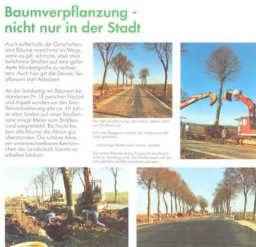
Figures 91: Luxembourg has transplanted 1,000 trees in recent years with a long-term success rate of 99%. One of the examples presented in the brochure "Straße und Umwelt in Luxemburg" (roads and the environment in Luxembourg) shows a road-widening scheme in which one row of trees is transplanted.
