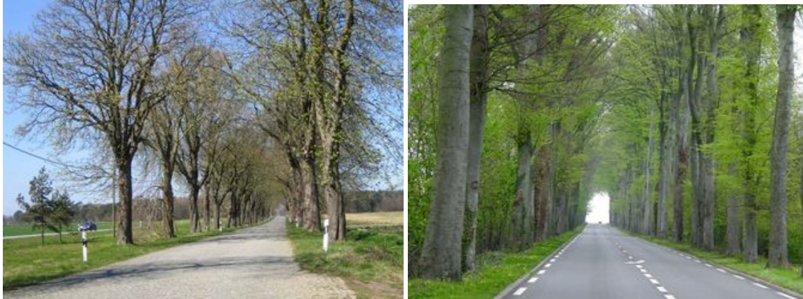
Figure 87: This historic road in Mecklenburg, retaining its original paving and its trees, is used for local traffic. Through traffic has been diverted onto a new road which runs parallel to the old one (on the left in the photo). Figure 88: On this Route Nationale (main road) in northern France, heavy goods vehicles travelling uphill use a parallel lane located beyond the avenue of tall beech trees.
