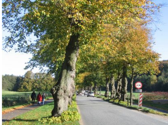
Figure 105: This double row of trees from 1830 (Rathlousdals Allé in Denmark) borders a roadway that is 5.1m wide, with traffic levels of 5,000 veh/day. It has been protected since 1979, and this is supplemented by a prohibition on winter salting, as is also the case in Freiburg in Germany. Elsewhere in Denmark screens are used to protect trees from the salt.
