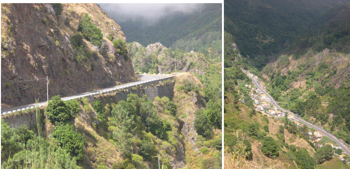
Fig. 68 and 69. Roads on the slope and at the bottom of a valley in Serra de Agua, Madeira, Portugal. (Photos by I. Español) A variety of road environmental effects should be taken into account. (Left) Short term effects: water aquifer reserves can be drained by the effect of road cutting at the base of the aquifer formation. (Right) Roads are an axis for human activity which must be taken into account by strategic planning.
