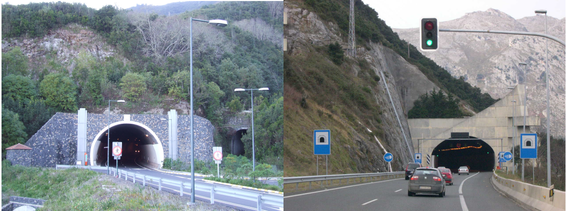
Fig. 43 and 44. Tunnel Mouths II. (Left) Structure covered by stone wall on the island of La Palma (Spain). (Photo by J.T. Rodríguez) (Right) Sophisticated ornamental walls for the Cantabrico Motorway (Spain). (Photo by I. Español) Note in both cases the slope above the tunnel's upper collapse which is partially integrated by the external structure design.
