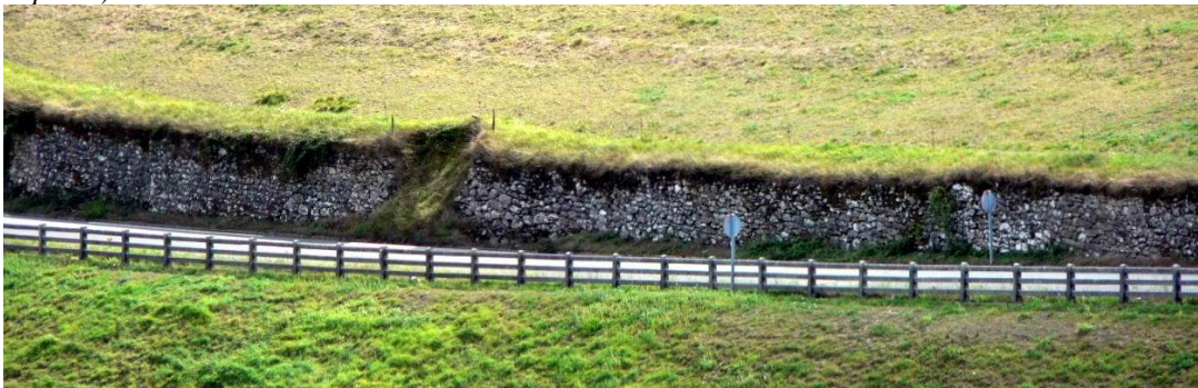
Fig. 25. A traditional stone wall works as a retaining wall for the road cutting, while the embankment has been successfully naturalised by grass. (Photos by I. Español)
