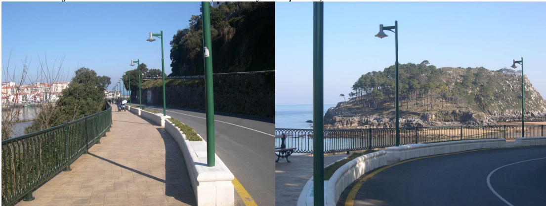
Fig.IV-10 and IV-11. (Left) Footpath separated from traffic lanes by a white parapet, including top gardening and lights. (Right) The footpath around the road bend includes a scenic viewpoint. (Photo by I. Español)
