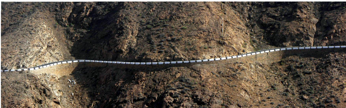
Fig. 80. Traditional character elements, such as a teeth- like safety barrier and retaining walls made from local stone, encourage a positive landscape integration. (Photo by I. Español).
