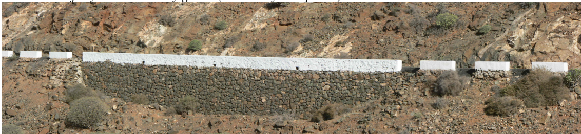
Fig. 26. The road platform is held by a retaining wall concealed under a finishing of traditional stone walling. Traditional stone walling and an old-fashioned white parapet provide a positive result in functional and landscape terms. (Photos by I. Español)
