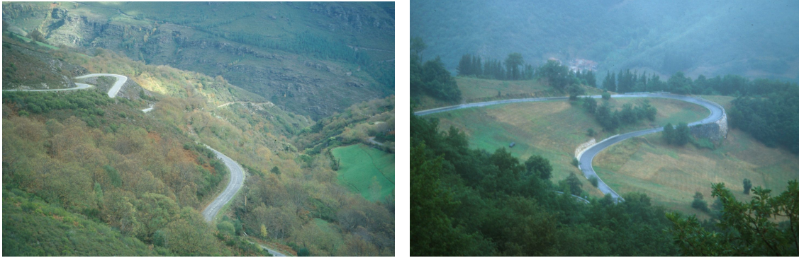
Fig. 10 and 11. Driving safely along hard alignments such as these steep and curved road shown in the pictures above, requires a better legibility of the road ahead, so tall vegetation has been removed at road verges. (Photo by I. Español)
