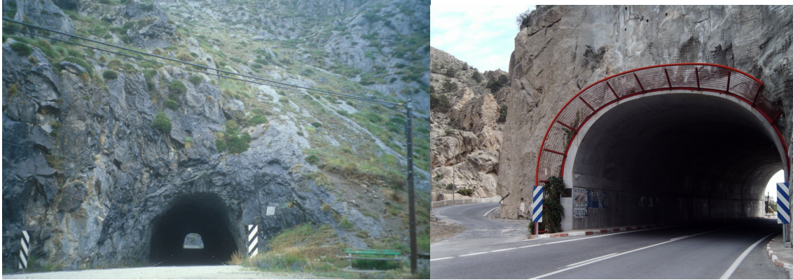
Fig. 41 and 42. Tunnel Mouths I. (Left) Carved tunnel for a one-lane road on the island of El Hierro (Spain). (Photo by I. Español) (Right) Red ornamental protection marquee and plastered rocks at a tunnel in Ricote Valley, Murcia (Spain). (Photo by L. Cruz)
