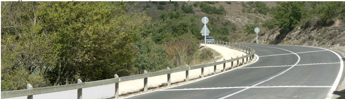
Fig. III-11. Speed reduction marks on the road and a low safety barrier create more footpath safety and comfort. (Photo by I. Español)
