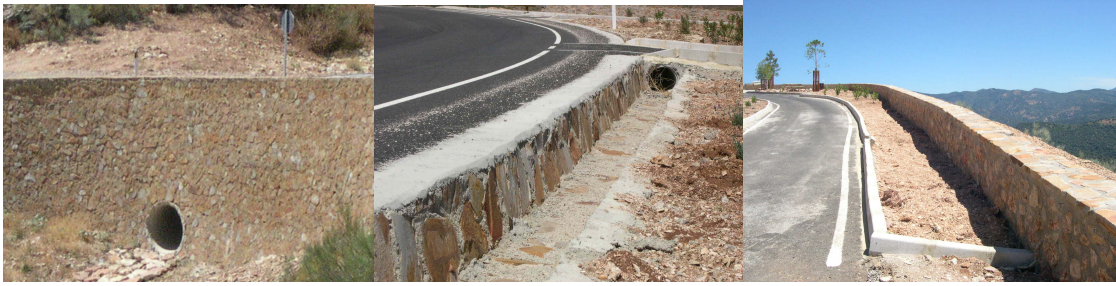
Fig. 60, 61 and 62. Sandstone is a consistent material which being used in different road elements (retaining wall, drains and parapets) builds up a sense of identity (Photos by I. Español).
