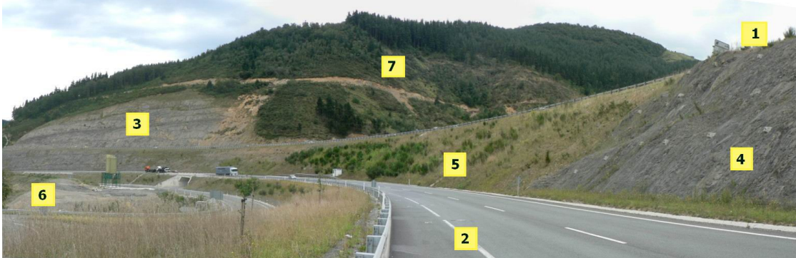
Fig. 76. Construction of a separated dual carriageway to expand capacity. (Photo by I. Español) Earthworks, particularly those of high- speed and high-capacity roads, determine road presence in
