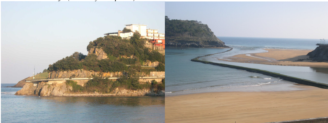
Fig.IV-4 and IV-5. (Left) The Karraspio road cut into the rocky slope. The cuttings of the main road to Ondarroa are noticeable above. Note the flying platform on the left. Sea is at high tide. (Right) The dam for the tide mill shows its alignment from Saint Nicholas Island to the river mouth at low tide. Note on the right of the picture the flying platform of the road to Karraspio. (Photo by I. Español)
