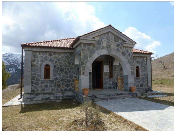
Picture 9 – Garni visitor centre (NW).
