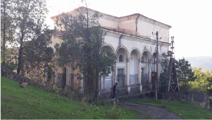
Upper station of the ropeway, 2015-16.
