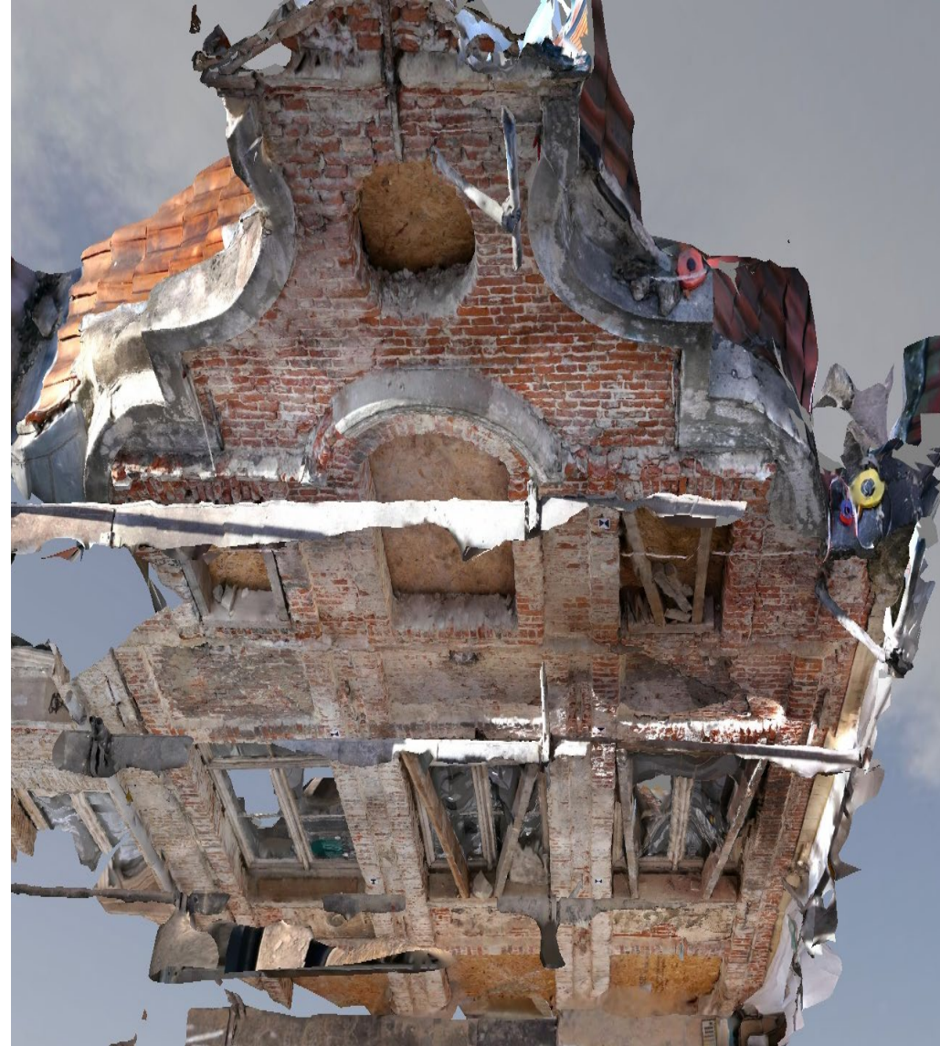
Photogrammetric capturing of a façade near the Grand-Place, Brussels
