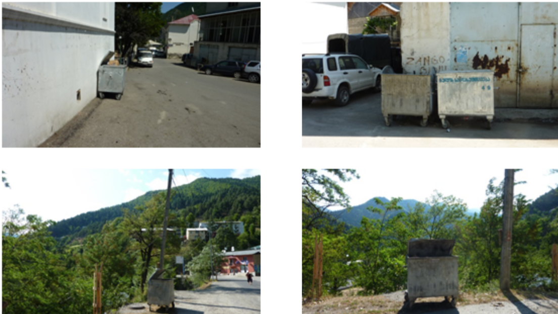
Figure 4 Examples of 1.1 m 3 steel containers used for primary waste collection
