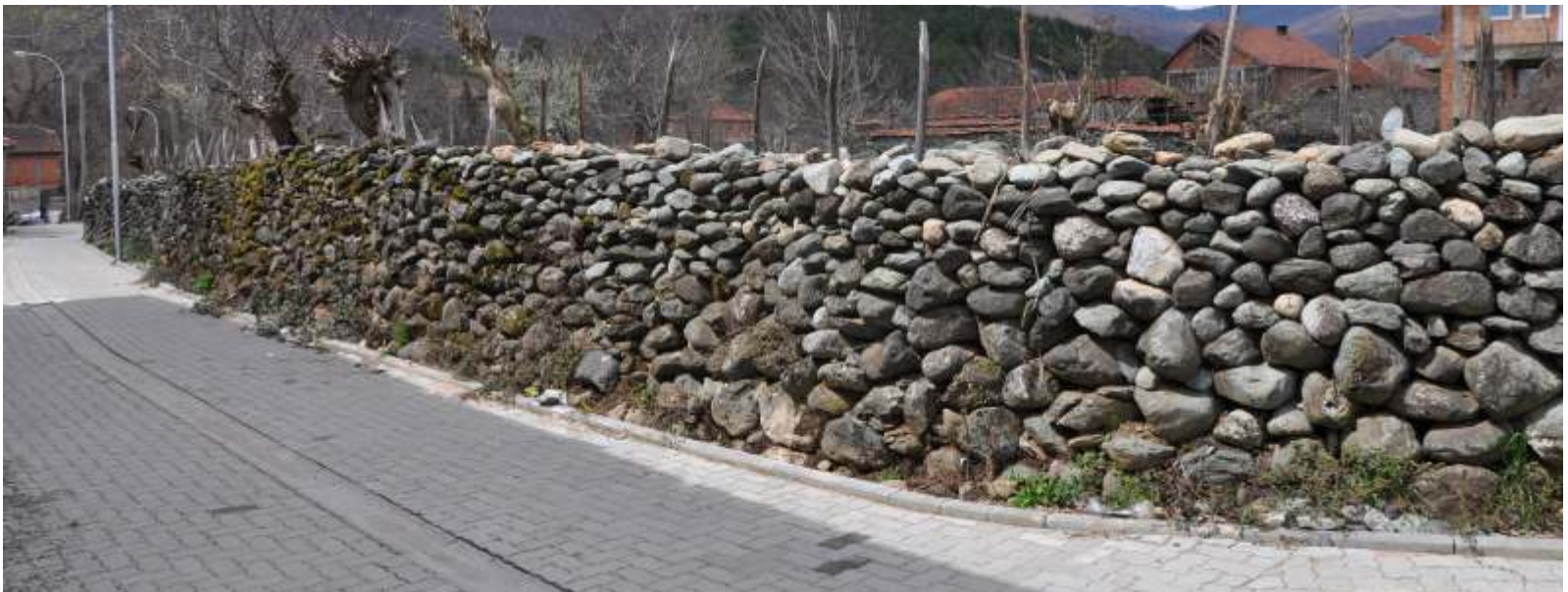
Wall built of river stone and wicker
