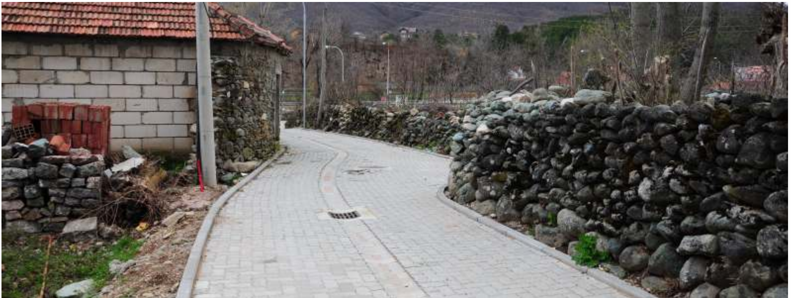
New pavement of the street with concrete slabs
