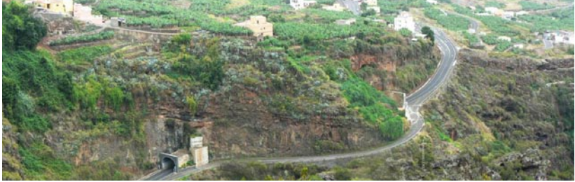
Photo 6. Environmental integration of tunnel and old road outlay in Los Galguitos (La Palma, Spain) (Photo by I. Español)
