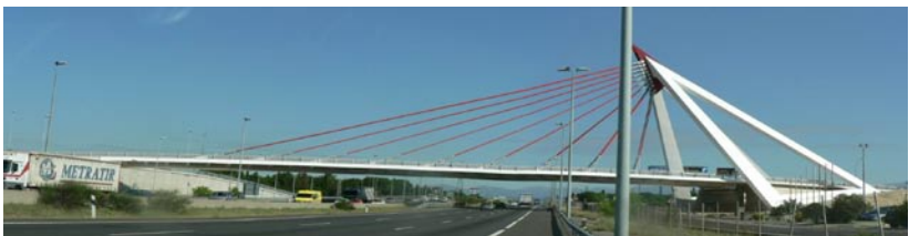
Photo 7. Bridge on the routinary urban A-6 motorway (Madrid, Spain) (Photo by I. Español)
