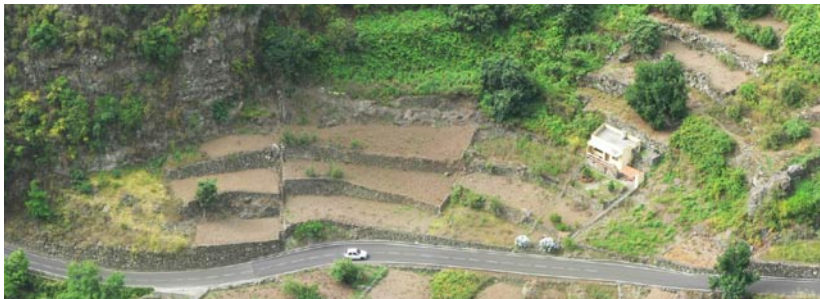
Photo 2. Road and agricultural terraces at Los Tiles (La Palma, Spain). (Photo by I. Español)
