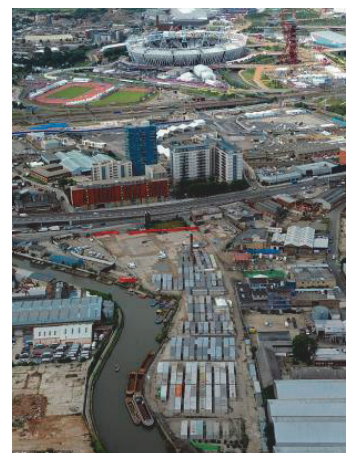
Poor conditions: The bad weather has left the site flooded with stagnant water, forcing the cleaners to use abandoned crates as makeshift 'stepping stones' to move around the site. This image shows how close the camp is to the Olympic Stadium
