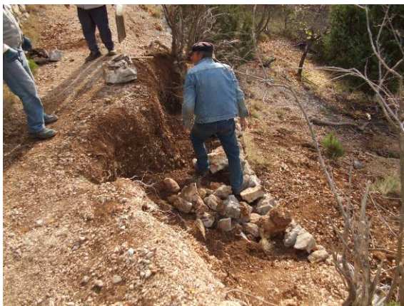
Renovation of traditional landscape elements in the surrounding, using traditional techniques and materials - pathways and drywalls (author: Vanja Kovačić)
