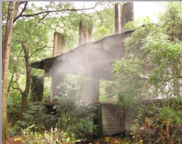
Ruin demolition and removal of invasive flora
