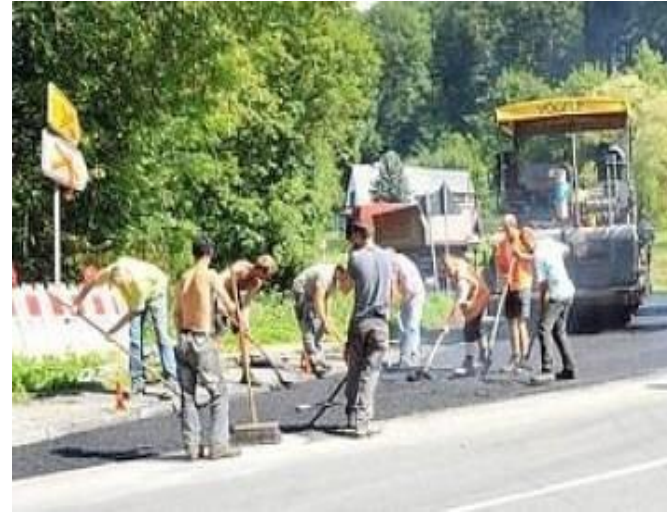
Germany - Rural road construction: 'typical' men's work
