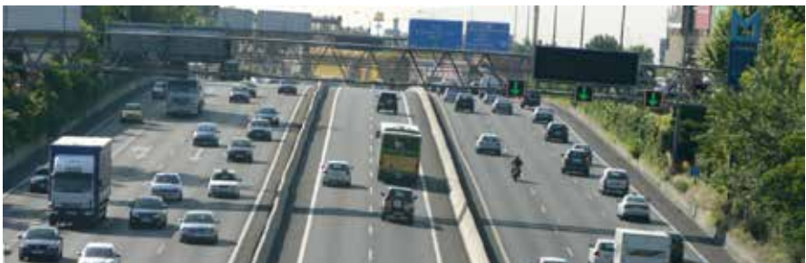
A6 urban motorway (Madrid, Spain)
