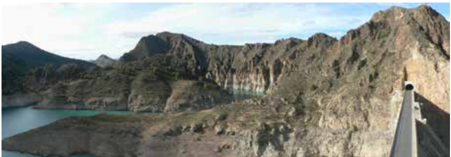
Cenajo dam and reservoir (Albacete, Murcia, Spain)
