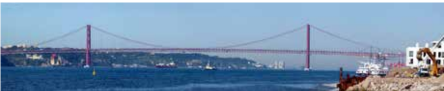
25th April bridge, Lisbonne (Portugal)
