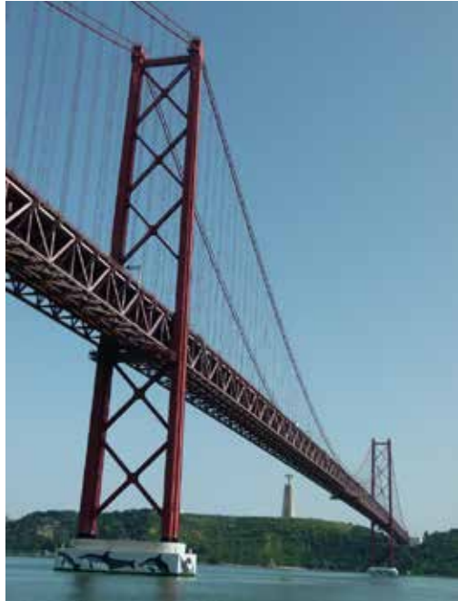
25th April bridge (Lisbonne, Portugal)
