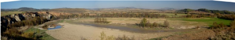
Figure 8: Post-restoration panoramic view
