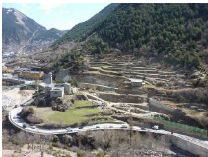
Figure 17: Works at the northern and southern entrances; beyond the building one can see the stone-walled terraces that characterise the landscape forming the background to the historical building
