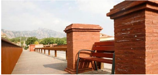
Figure 6: Bridge over the Torrent de l'Illa at El Bruc
