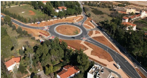
Figure 4: Junction improvement in roads BV-1221 and BV-1275
