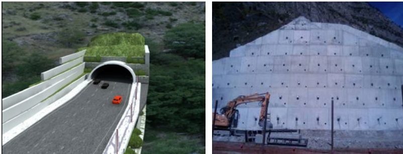
Figure 9: On the left the photomontage of the final appearance of the south entrance to the Túnel de la Tapia; on the right a segmental wall of similar dimensions built in another part of Andorra
