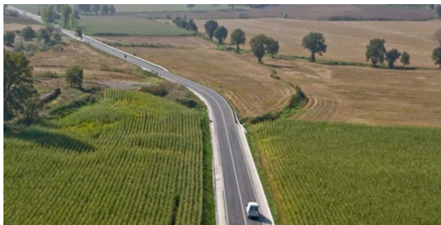
Figure 2: Route improvement in C-153 road
