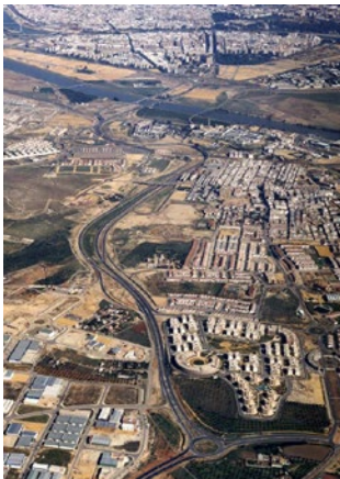
Figure 5: A road structure orders space in the metropolitan area of Seville
