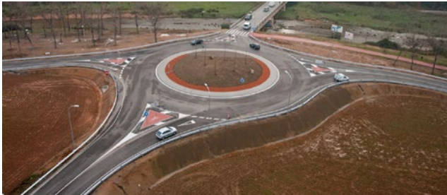
Figure 3: Junction improvement in road BV-1433
