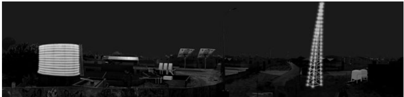
Figure: A view of Benquerencia Industrial Estate from the high-speed train, with “spotlight” intervention
