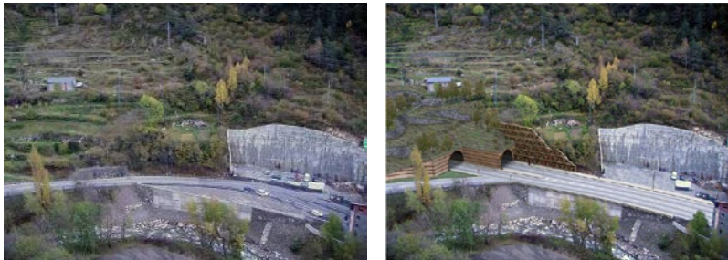
Figure 15: South entrance, initial stage
